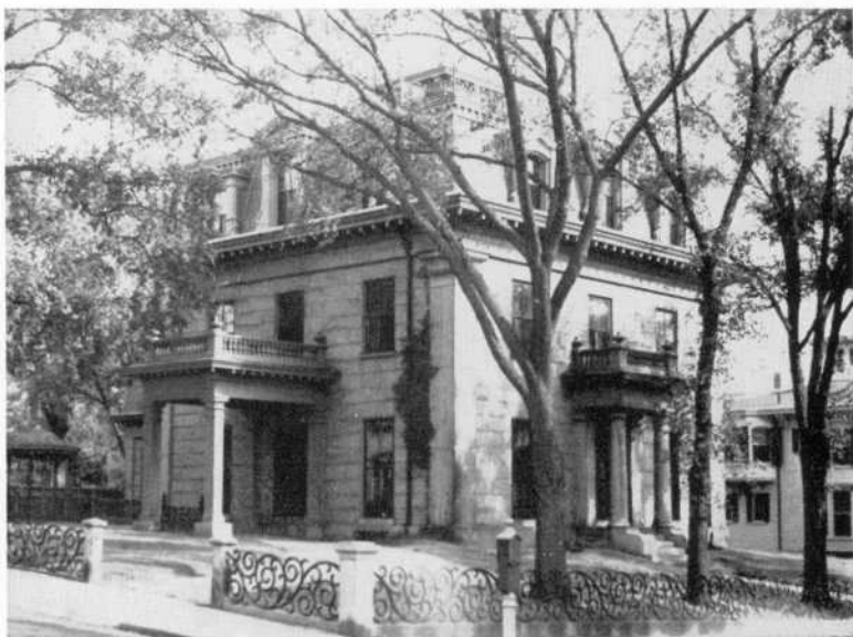
FALL RIVER HISTORICAL SOCIETY BUILDING Formerly on Columbia Street
