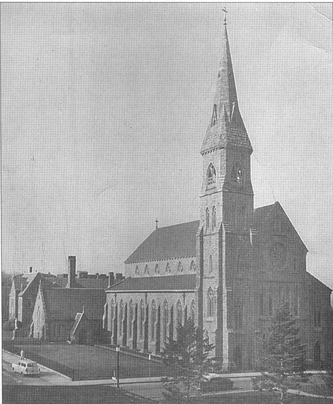
Left, the Fall River Historical Society is one of many examples of granite buildings that can be found throughout the city. Above, St. Mary's Cathedral is built with Fall River granite in an 11th-century Gothic style. Fall River granite was also used to build mansions in Newport, R.I., parts of Fort Adams and the base of the Statehouse in Albany, N.Y.
